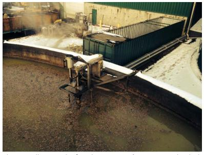
clients cannot use floating pontoons in their installations. The fact that VaraCorp's aerator can be dock or wall mounted using a mounting bracket supplied by VaraCorp is a plus for these companies.
